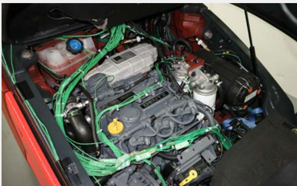
Fig. 7: The temperature and pressure sensors are installed in the specified locations in the engine compartment. The green cabling shows routing of the Type K thermocouple sensors to the measurement modules located outside the confined engine compartment.
